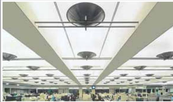
40" diameter indirect bowl, suspended by concealed aircraft cable and illuminated by compact fluorescent lamps.
