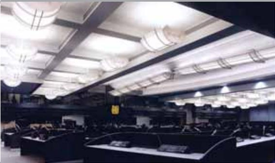
Custom, direct/indirect pendant luminaires utilize a 4' wide x 5' long 'barrel' design with opal acrylic shroud and perforated end plates that are illuminated by T8 dimmable fluorescent lamps.
