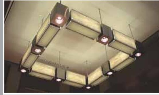
This 14'x14' structure combines the use of polished metals and alabaster acrylic and is illuminated by a combination of T5HO and MH PAR lamps.
